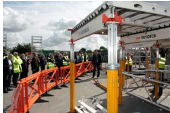
External and Internal Advance Guardrail demonstrated on Aluminium Towers
