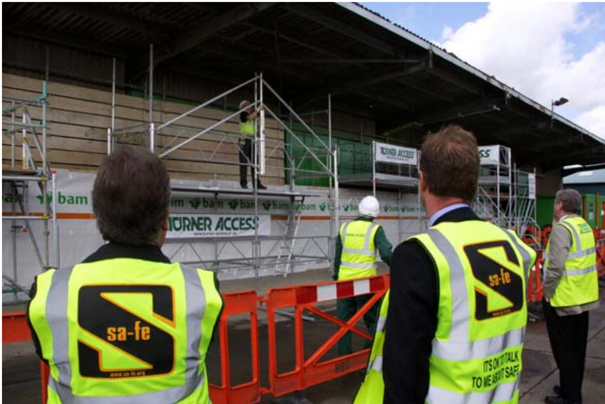
External Telescopic Advance Guardrail demonstrated on System Scaffolding
