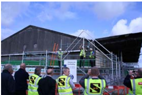
External Telescopic Advance Guardrail demonstrated on Tube and Fittings
