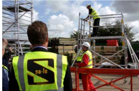
External and Internal Advance Guardrail demonstrated on Aluminium Towers
