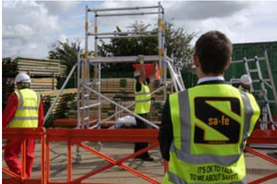
External and Internal Advance Guardrail demonstrated on Aluminium Towers
