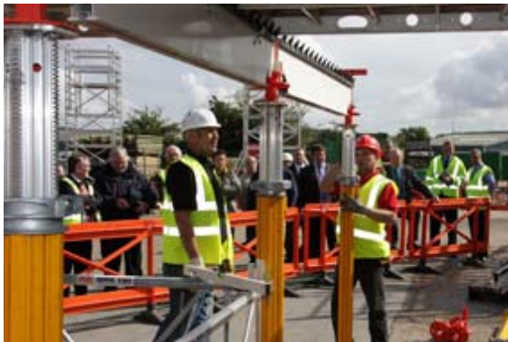
Falsework erected from the ground to avoid work at height
