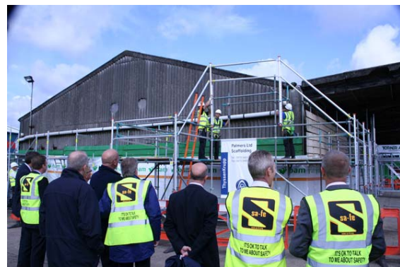
External Telescopic Advance Guardrail demonstrated on Tube and Fittings
